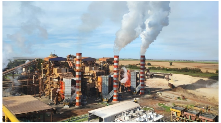
Aerial view of boilers nº 1, 2 and 3
